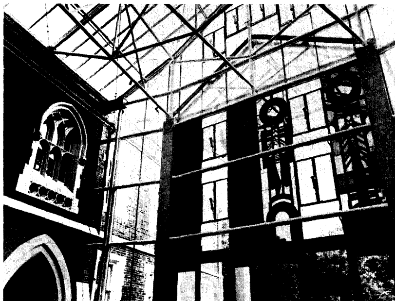
Glass installation at the front of the atrium, where it meets the cloistered wall of the old building.
